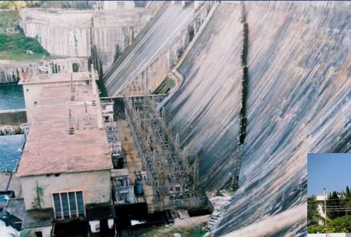
Power generation at main dam Badra KNNL India
