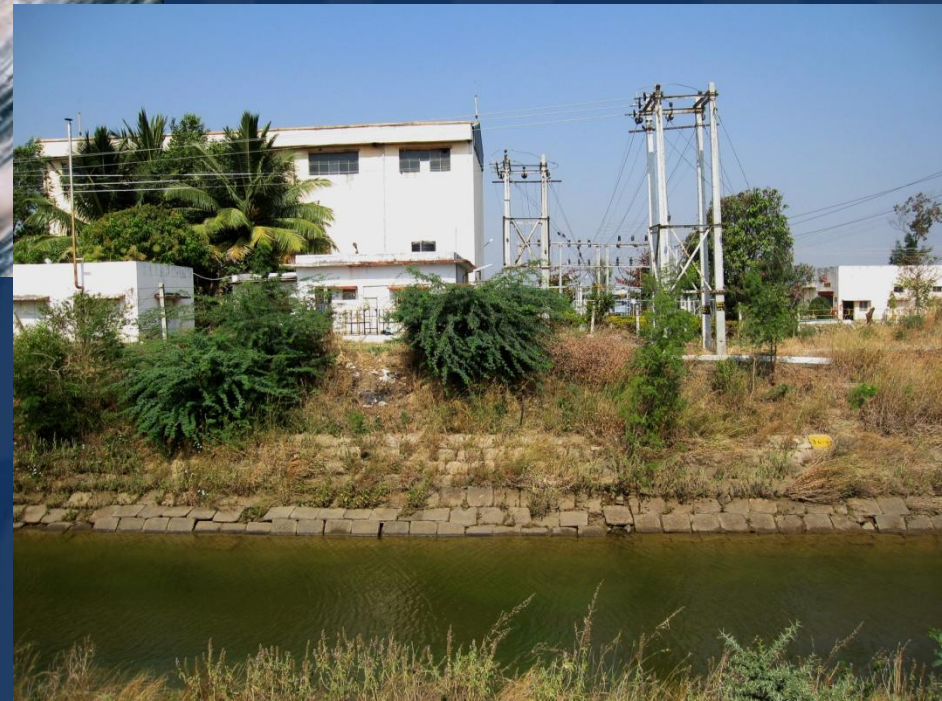
Power generation unit along a Canal Naryanpur Karnataka India
