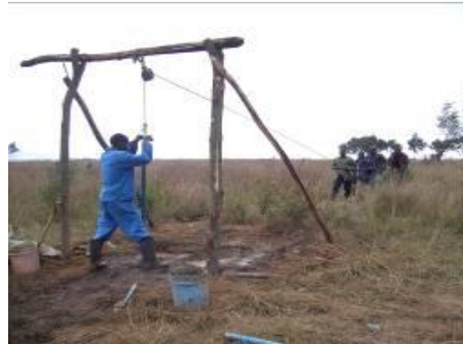
Photograph 2. Manual drilling a 30 m borehole using Baptist drilling (Soil: compact clay, time taken: 3 days)
