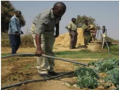
Photograph 1. Hand Digging a small diameter well of 20 m deep, using a “well ventilator”
