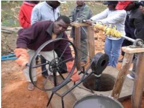
Photograph 1. Hand Digging a small diameter well of 20 m deep, using a “well ventilator”
