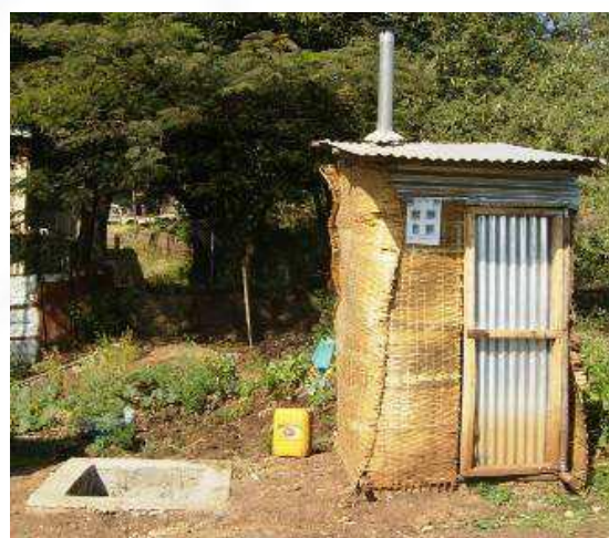
Figure 4. Fossa alterna with organic woven superstructure, Arba Minch 4 .
