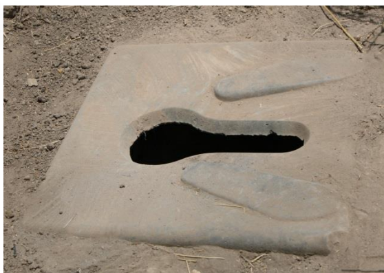
Figure 5. Close up of Arborloo slab, East Arsi.
