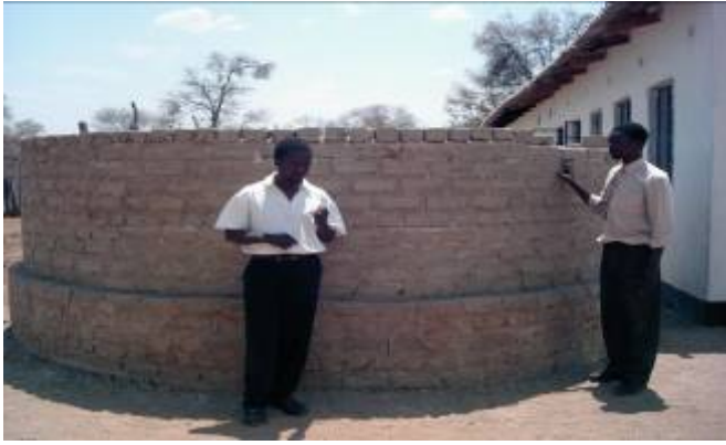
Figure 3: Roof top rainwater harvester under construction in Tsholotsho district
