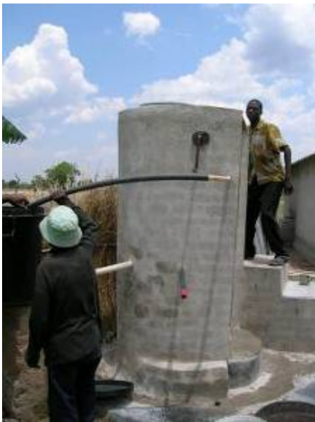
Figure 11: Rope pump with several outlets, potentially for in-house connections, Marondera district
