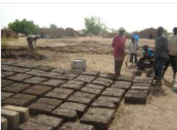
Photo 7: Brick moulding at the site of one of the dams developed by Plan Ghana.
