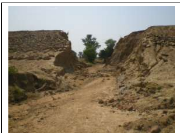
Photo 6: Breached dam wall of a small reservoir in Upper East Region. Photo: Eric Ofosu
