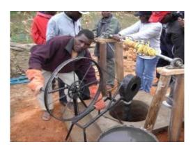
Photograph 1. Hand Digging a small diameter well of 20 m deep, using a "well ventilator"
