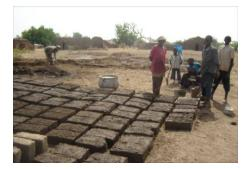
Photograph 4. Brick moulding at dam site
