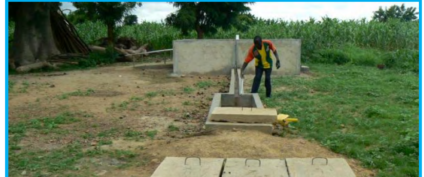
Burkina Faso: a borehole fitted with hand pump and water troughs- very common in West Africa.
