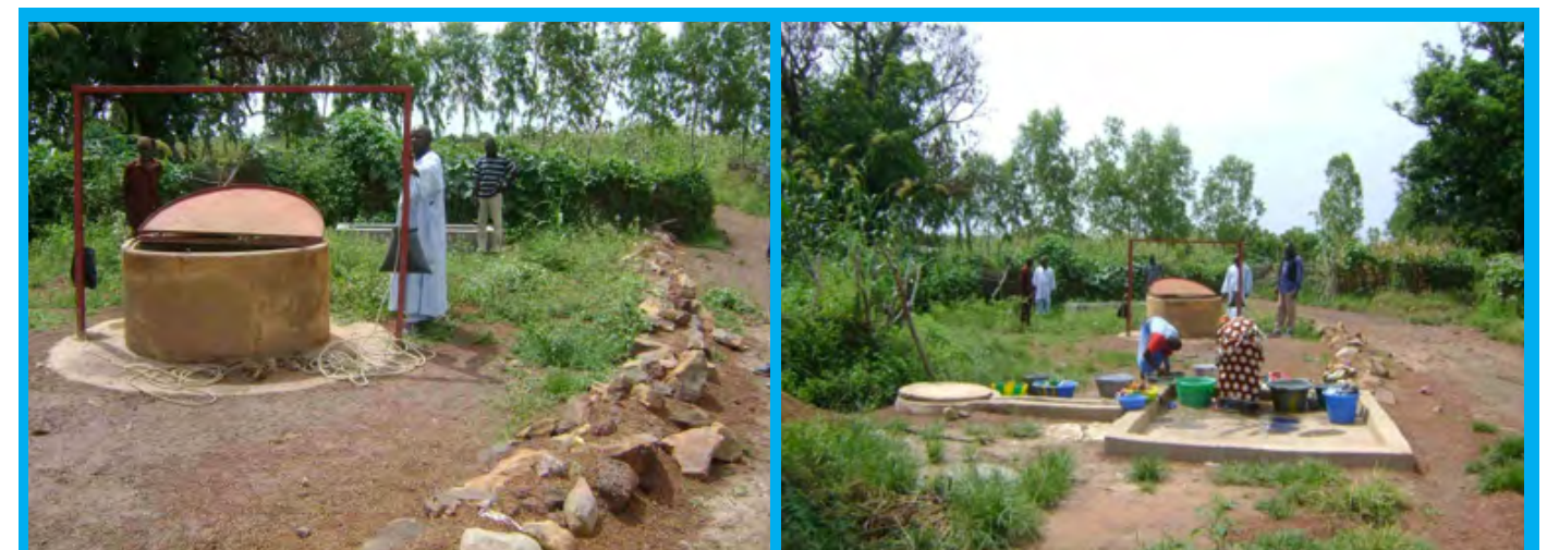
Mali: a large diameter well rehabilitated in Bablebougou with a washing area for women and troughs for cattle. This well has helped in reducing the pressure on the village borehole for better sustainability.
