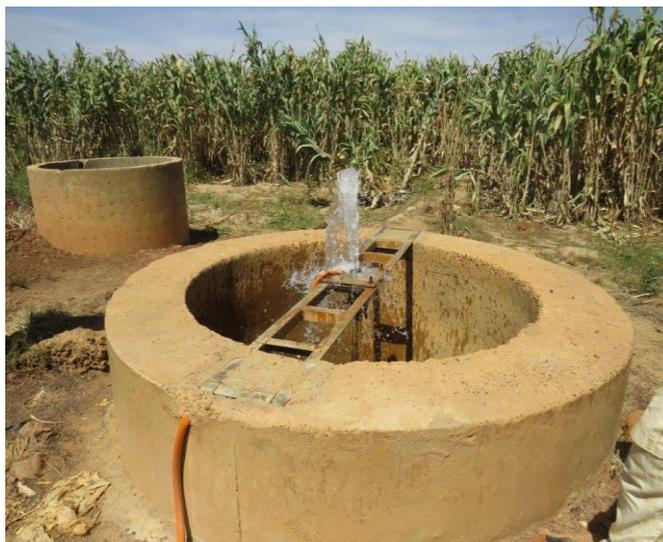
Figure 1 Water well functioning through solar power, Bambeye, Tahoua Region, Niger. Photo taken by Cecilia Benda (Nov 2019)
