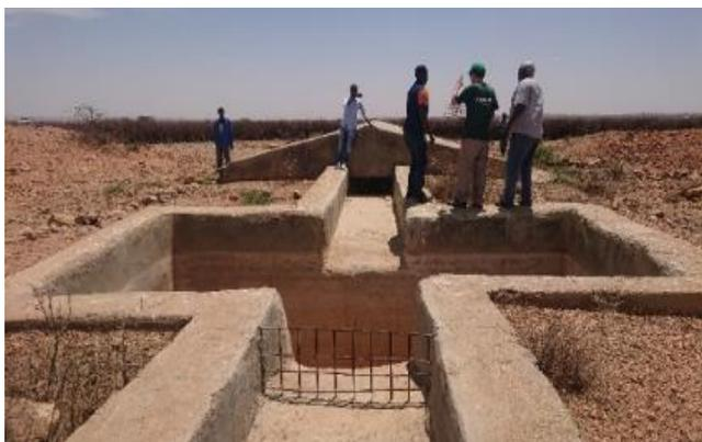
Figure 7 - Berkhads are cemented reservoirs to collect rainwater that when combined with a system of filters or household water treatment products can provide water for drinking, washing and other domestic uses, mainly during the dry season. Photo taken by Martin Findlay (April 2019).
