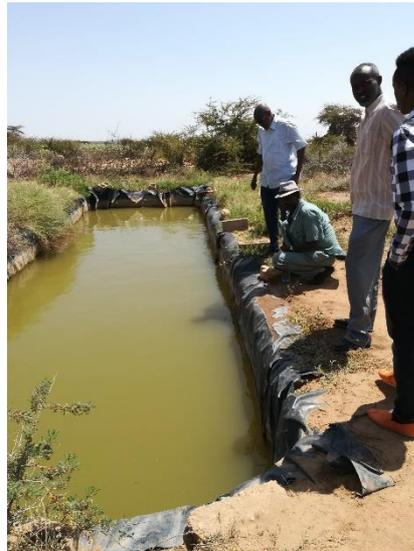
*Figure 9 - Water basins lined with plastic sheet with (left) or without (right) cover (to reduce evaporation). These structures are located beside tree orchards or gardens and provide water for irrigation during dry spells or the longer dry season. Photo taken by Cecilia Benda (2014).*
