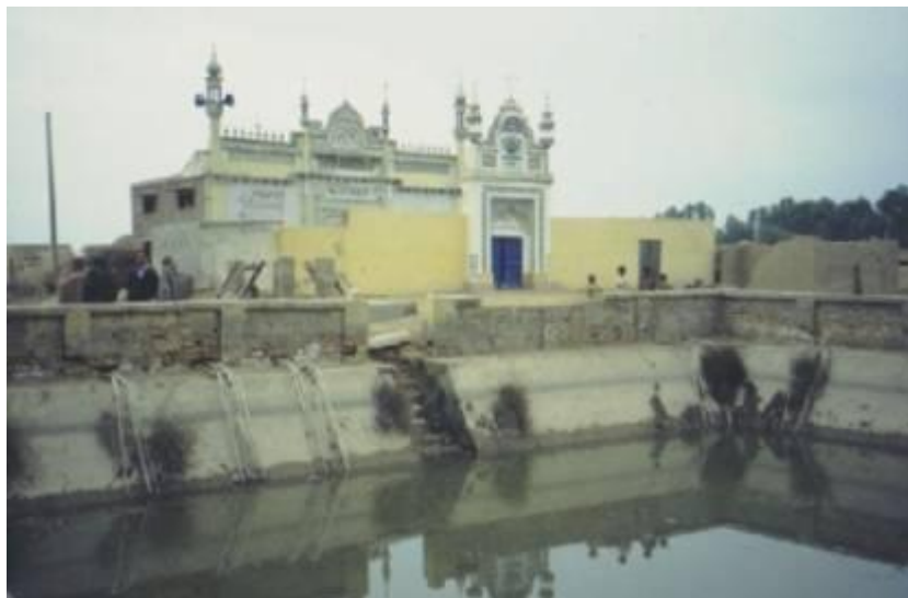
Photograph 3. Open reservoir filled with water from irrigation canals in Hakra 6R, Punjab, Pakistan. The water is heavily polluted during transport and storage in the tank that often serves as solid waste collector as well (Ensink et al. 2002; van der Hoek et al. 2002). The pipes lead to individual houses where an electric pump provides the pressure necessary to serve the entire house. The water flowing from the tap looks clear and gives a false impression of good quality.
