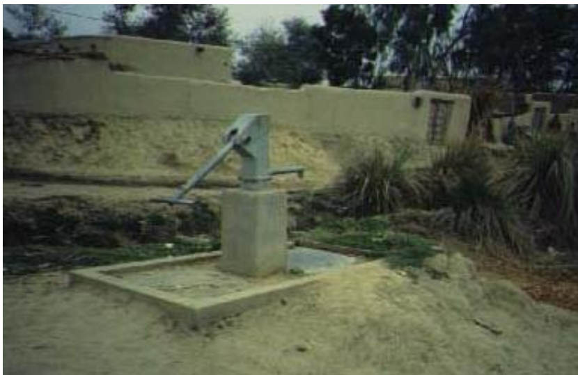
Photograph 5. In arid regions of South Asia and North Africa, pumps and wells are often dug near unlined irrigation canals to benefit from the local groundwater recharge. While seepage from canals reduces irrigation efficiency, this indirect multiple use of water may have health benefits, such as here in Hakra 6R in Punjab, Pakistan, where the groundwater is too saline for consumption. The horizontal filtration through the soil generally improves the canal water (Boelee et al. 2007; Ensink et al. 2002; Meijer et al. 2006; Shortt et al. 2003, 2006).
