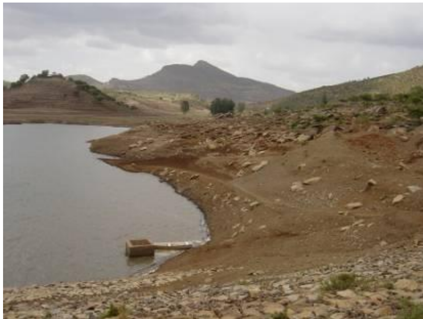
Photograph 15. Catchment management is important for springs, wells and rain water harvesting structures such as this small reservoir Mai Negus in Tigray Region, northern Ethiopia, to reduce erosion and siltation as well as pollution by grazing livestock and runoff. Such measures can improve the water quality and reduce the need for treatment (Million 2008).
