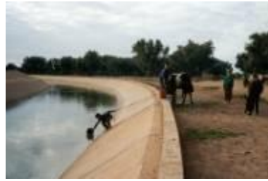
Photograph 14. Children hazardously collecting water from large irrigation canal in Tessaout Amont, Morocco. Several children and even adults drown in this canal every year. Though it doesn't show on this particular day, the water can flow very fast and wipe you away easily while it is very difficult to get out.
