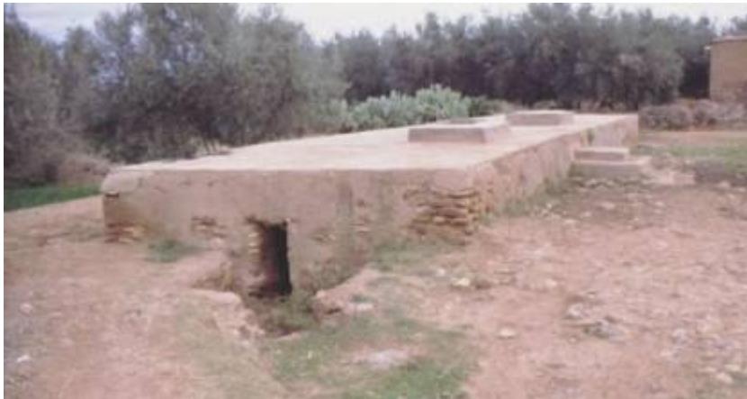
Photograph 12. Communal tank, old stone structure rehabilitated with cement in Tessaout Amont irrigation system in central Morocco (Laamrani et al. 2000). Farmers use part of their irrigation water allocations to fill it. What looks like a door is the intake and the manholes on top are used to haul water out. Before it gets into the tank, the water is transported over some 15 kilometres: first from the reservoir through the old riverbed, then into cement-lined main canals and elevated concrete secondary canals system all the way to the site. The last 10 meters it flows over the ground by the side of the road and gets polluted by animal droppings and other waste.
