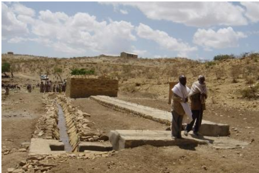
Photograph 7. Multipurpose water system in Adidaero, Tigray Region, Ethiopia: left an irrigation canal, right a horizontal filtration gallery for clean drinking water (Ebato and van Koppen 2005). It took several months before the community accepted the water as clean water for consumption – the convincing argument being a field worker who drank the filtered water instead of buying bottled water.
