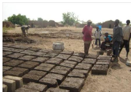
**Photograph 4. Brick moulding at dam site**
