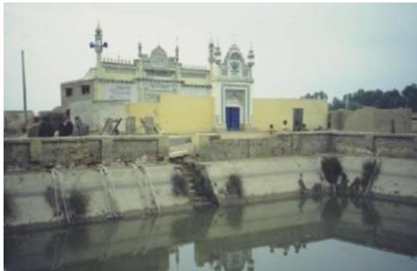
**Photograph 3. Open reservoir filled with water from irrigation canals in Hakra 6R, Punjab, Pakistan. The water is heavily polluted during transport and storage in the tank that often serves as solid waste collector as well (Ensink et al. 2002; van der Hoek et al. 2002). The pipes lead to individual houses where an electric pump provides the pressure necessary to serve the entire house. The water flowing from the tap looks clear and gives a false impression of good quality.**
