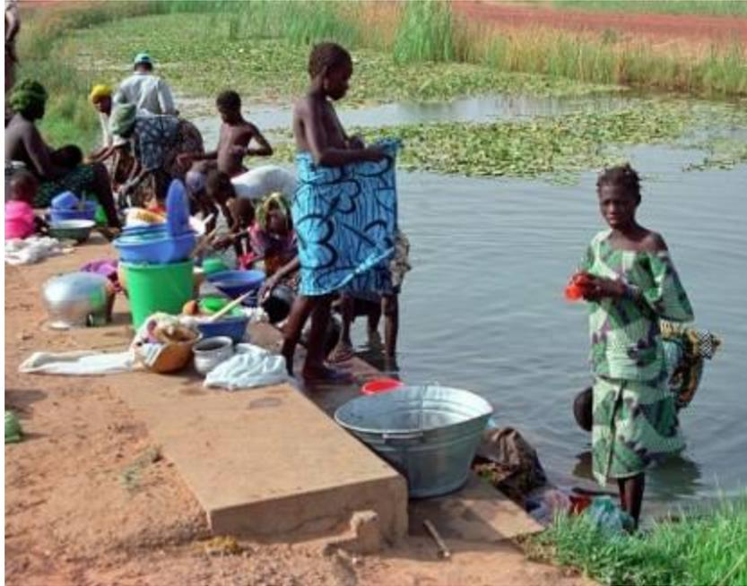
**Photograph 11. In many large-scale irrigation systems, steps have been built on large canals to facilitate access to the water for domestic purposes such as bathing and laundry. While this reduces the drudgery of water collection, it may also expose people, especially women and children, to schistosomiasis, such as here in Office du Niger irrigation system in Mali (Boelee and Madsen 2006).**
