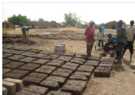
**Photograph 4. Brick moulding at dam site**
