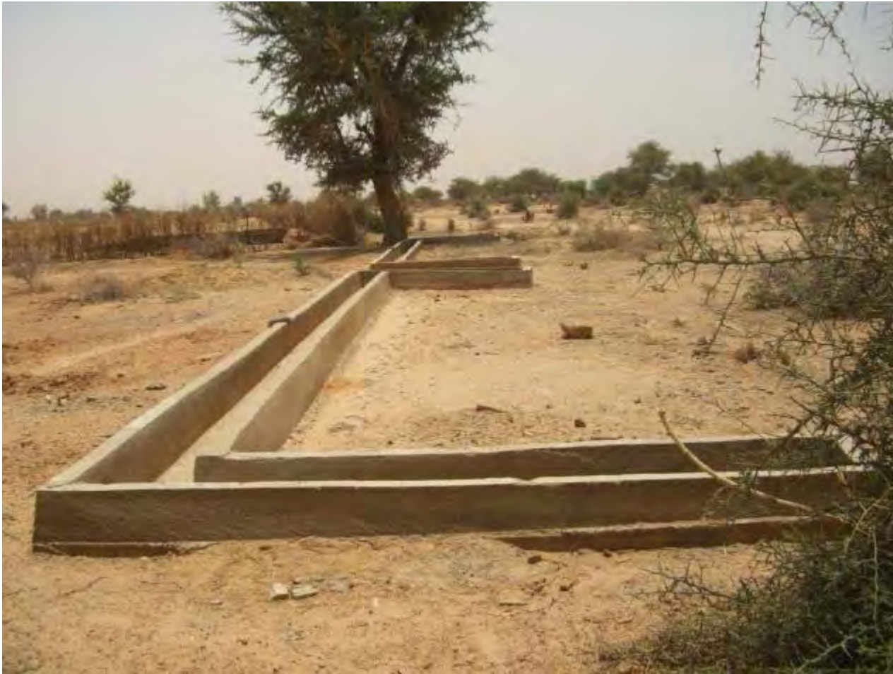
Soumatte cattle trough underconstruction
