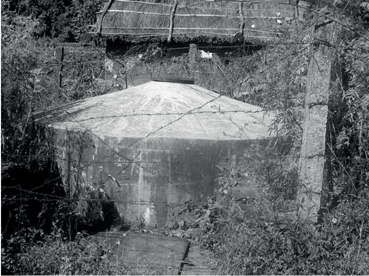
Figure 5.2 25,000 liter Mul Pani drinking water tank
